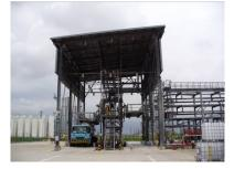
load all manholes on the truck top without the need to move the vehicle.
