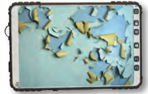
Tank lining delamination image as displayed on tablet
